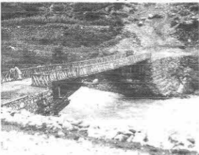
Passage to India. This bridge, a fine example in the use of local materials is sturdier than most. The water it spans is at a low level, though fast moving. Later in the year as the level rises the local children will not have the opportunity to take in the scenery. The photograph was taken in the Kaghan Valley.
